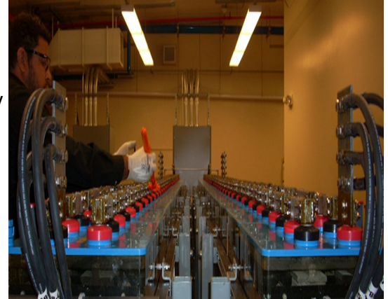
SPS installing UPS Flooded Battery System
